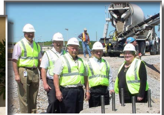
R-L Commissioner Janice Thomson and Lew Holloway are joined by employees of the Niagara Falls Bridge Commission on the construction site of Phase Two.
